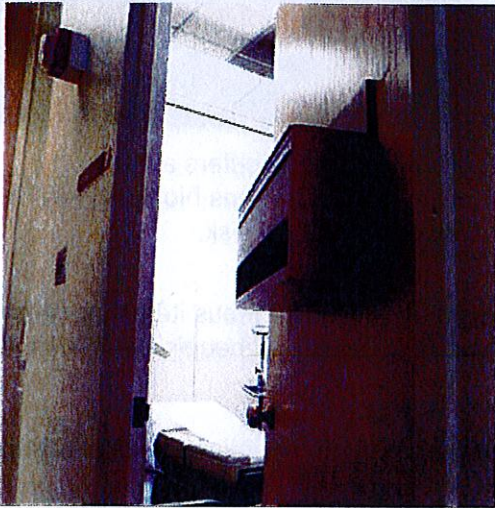
Figure 14: Chart box affixed to an examination entrance door, which protrudes over 4 inches.
