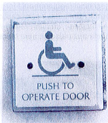
Figure 4: Automatic door opener, with large push button.
