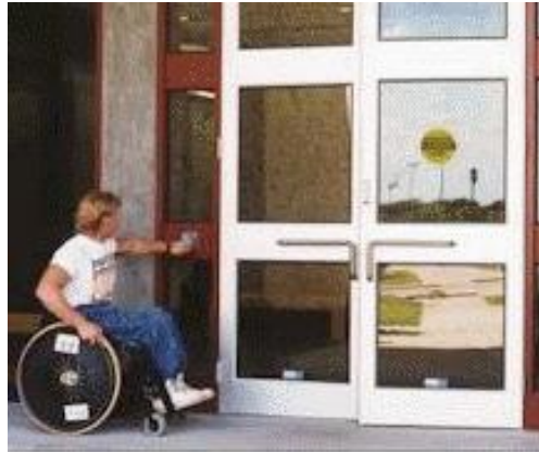
Figure 5: Automatic door opener, with large push button affixed to left of sliding doors.
