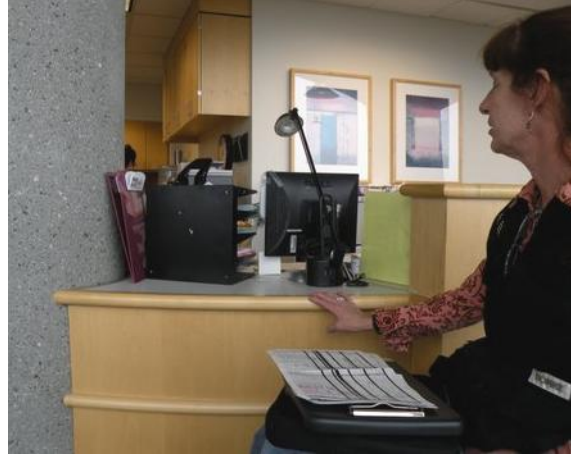
Figure 17: Computers and miscellaneous items block access to lower reception desk.
