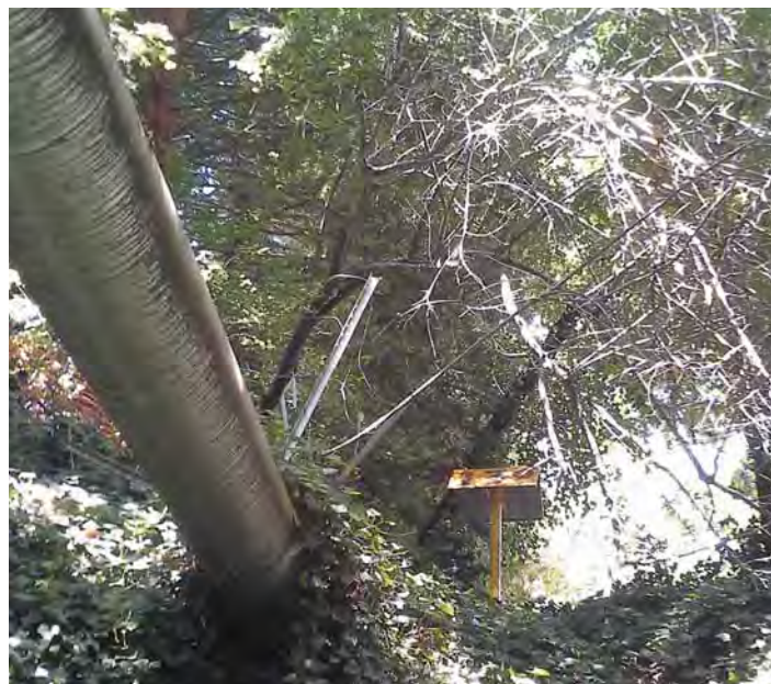
The San Jose line inside protective sleeve traveling above ground across a seasonal stream along the Iron Horse Corridor.
