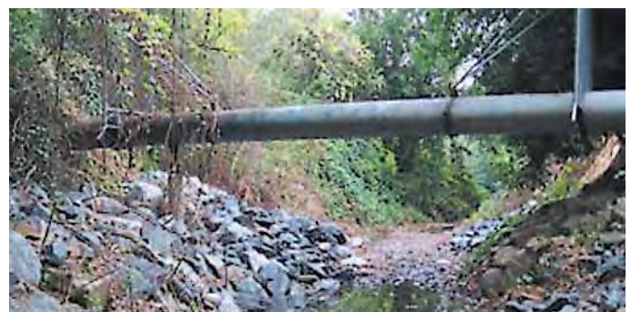
Examples of other pipelines crossing steam areas in California and Washington States.
