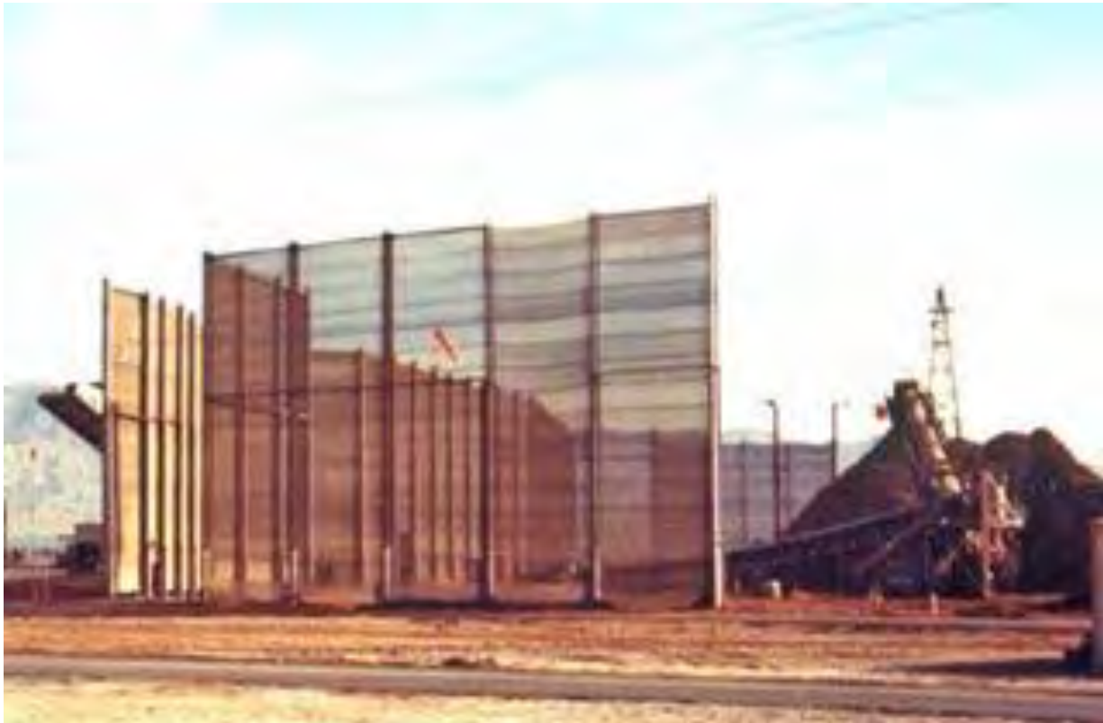
Figure II-1: Typical Wind Screen - constructed to protect a down-wind stockpile.
