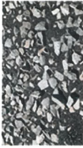
Coal dust in ballast section
