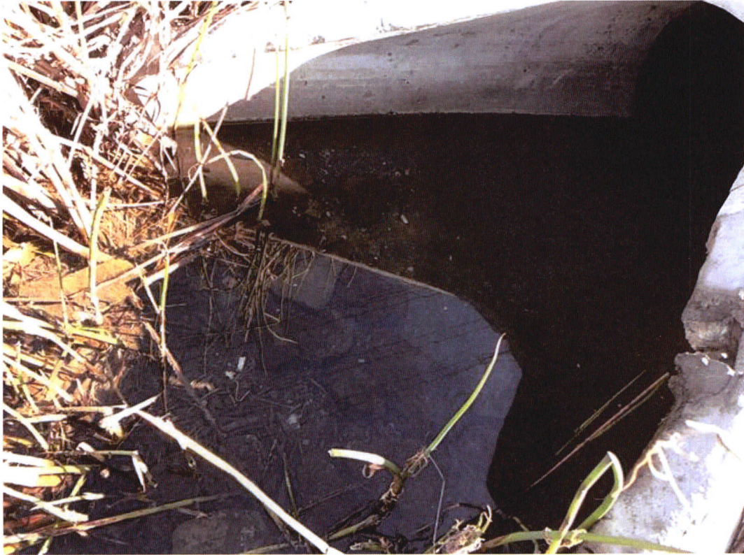
Photograph 2. The Outfall (Location A). February 28, 2017.
