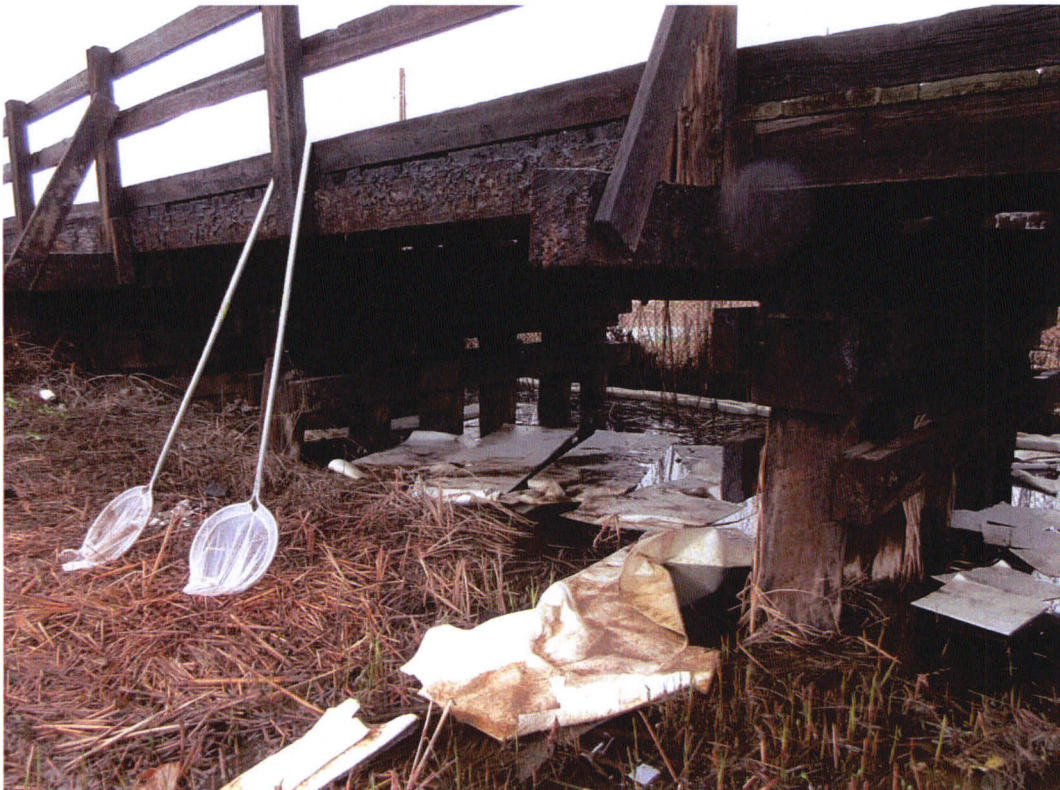
Photograph 10. Under the Burlington Northern Santa Fe Bridge (Location C). February 4, 2017.
