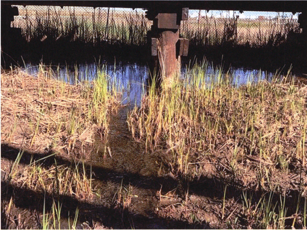
Photograph 5. Post Boom and Dam Removal (Location C). February 28, 2017.
