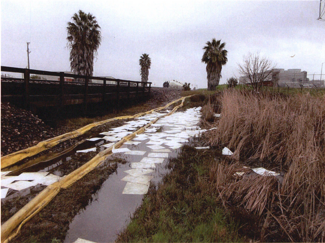
Photograph 9. The Burlington Northern Santa Fe Bridge (Location B). February 6, 2017.
