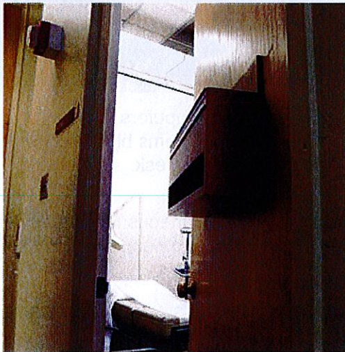
Figure 14: Chart box affixed to an examination entrance door, which protrudes over 4 inches.
